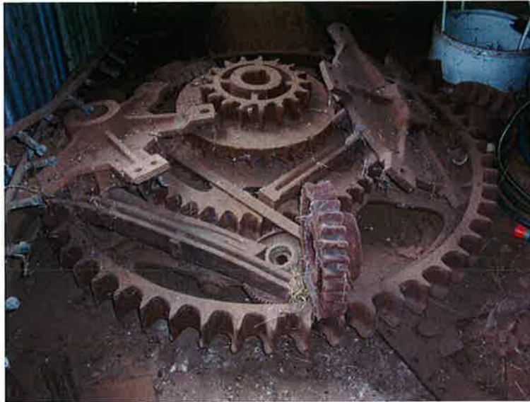
Worn out gears that have been replaced.
